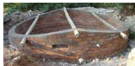
The bricked reservoir is 2m deep
